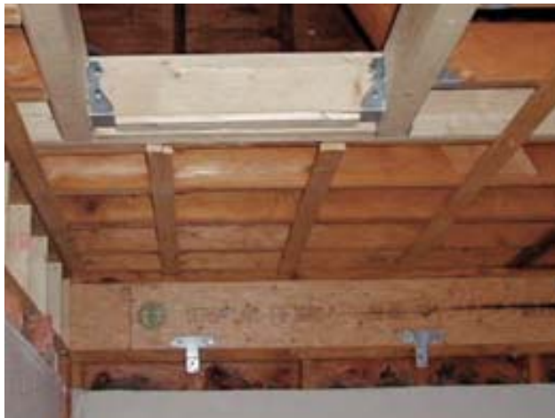
Figure 5. T-straps tie the LVL beam to the original plate at 16-inch intervals, helping to prevent the beam from rolling outward under lateral loads.
