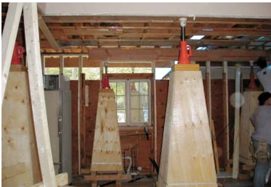
Figure 3. Site-built pyramidal jacking stands safely extended the screw jacks' reach to just below the lifting beams.
