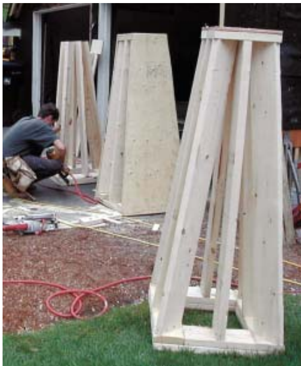
Figure 3. Site-built pyramidal jacking stands safely extended the screw jacks' reach to just below the lifting beams.
