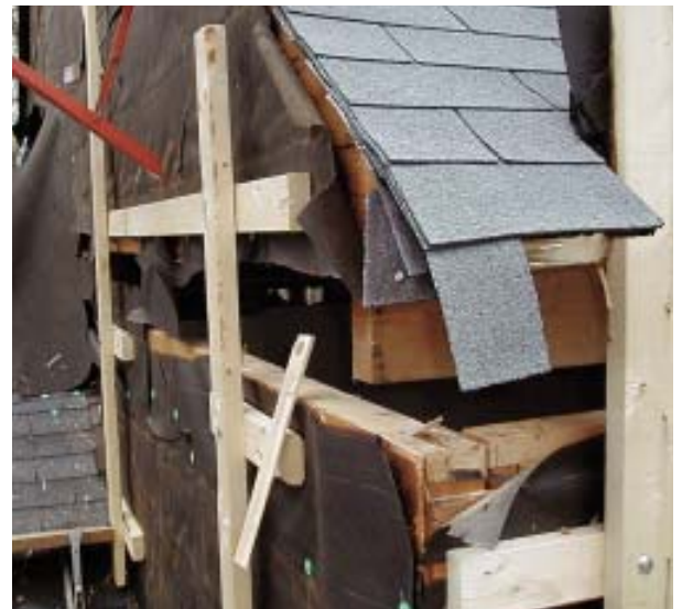
Figure 2. To maintain the original alignment and prevent the roof structure from shifting during lifting, the author's crew bolted 2x4 vertical struts to the tops of the walls around the house's perimeter.
