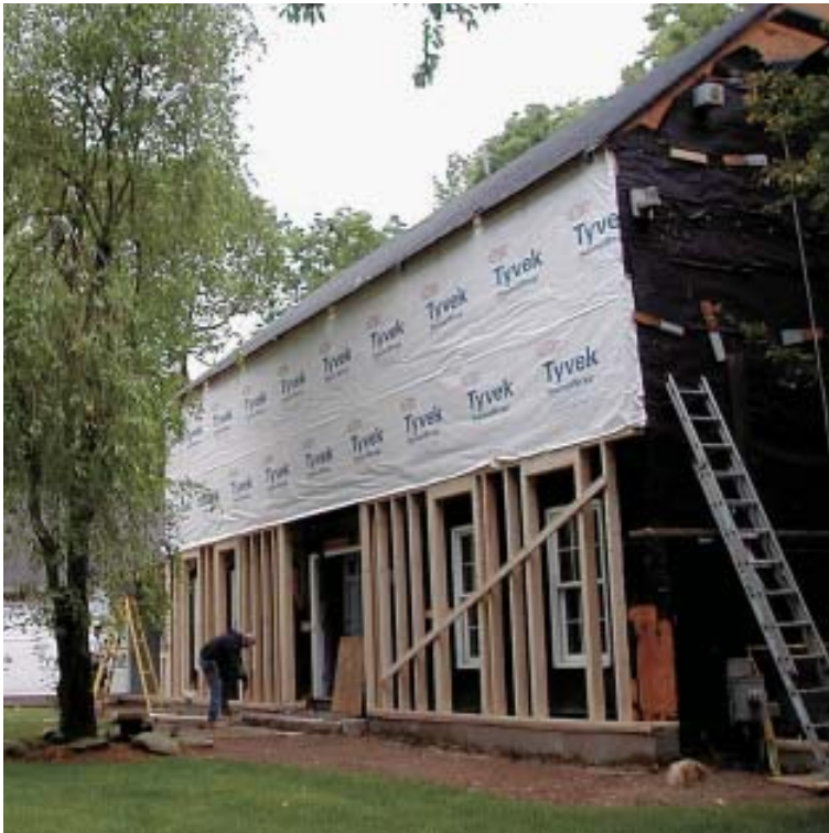
Figure 10. While the front wall went up quickly to support the building at its new height (left), the center and rear partitions had to be revised one stud at a time, by cutting and sistering in full-length studs under a new top plate. Nonbearing interior partitions were elevated with short cripple-wall sections (below).
