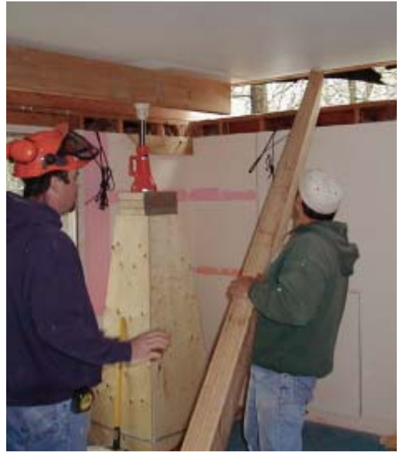
Figure 4. Working in small increments, the seven-man crew slowly raised the roof structure by 9½ inches, allowing the nominal 4x10 engineered LVL plates to be inserted into position on top of the wall.
