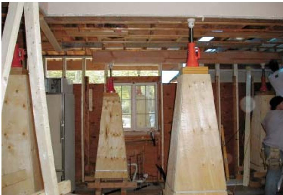
plywood and screwed it with  $1\frac{5}{8}$ -inch galvanized deck screws. As a final precaution, we wrapped a band of perforated, galvanized-steel strapping around the base about 8 inches up from the bottom and screwed through it into the studs with  $2\frac{1}{2}$ -inch galvanized deck screws. In the unlikely event one or more studs failed under load, we figured the band would help keep the base from spreading.
