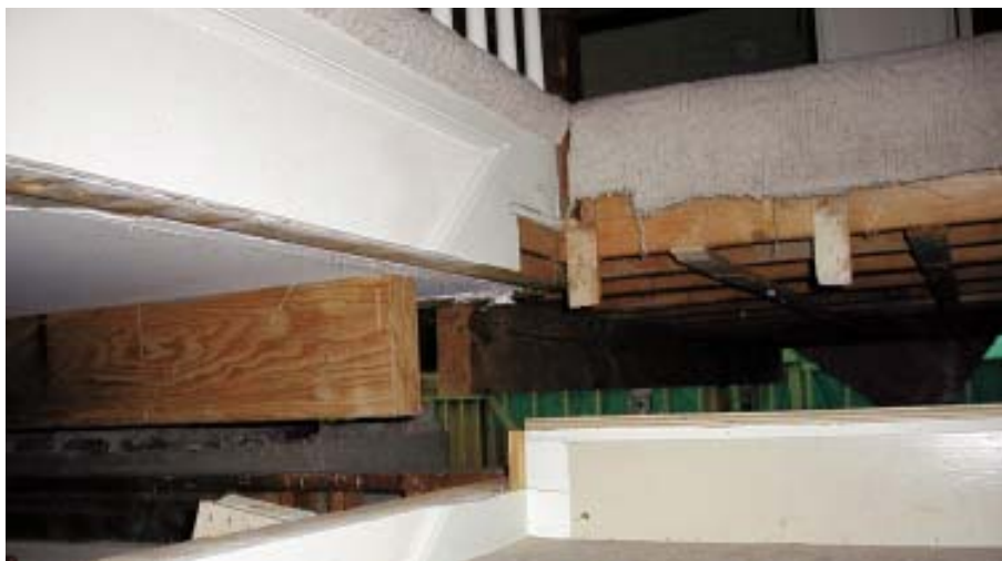
Figure 6. Though the staircase would be rebuilt, the original stair helped determine the distance that the first-floor ceilings were raised: two riser heights, or 15 inches.
