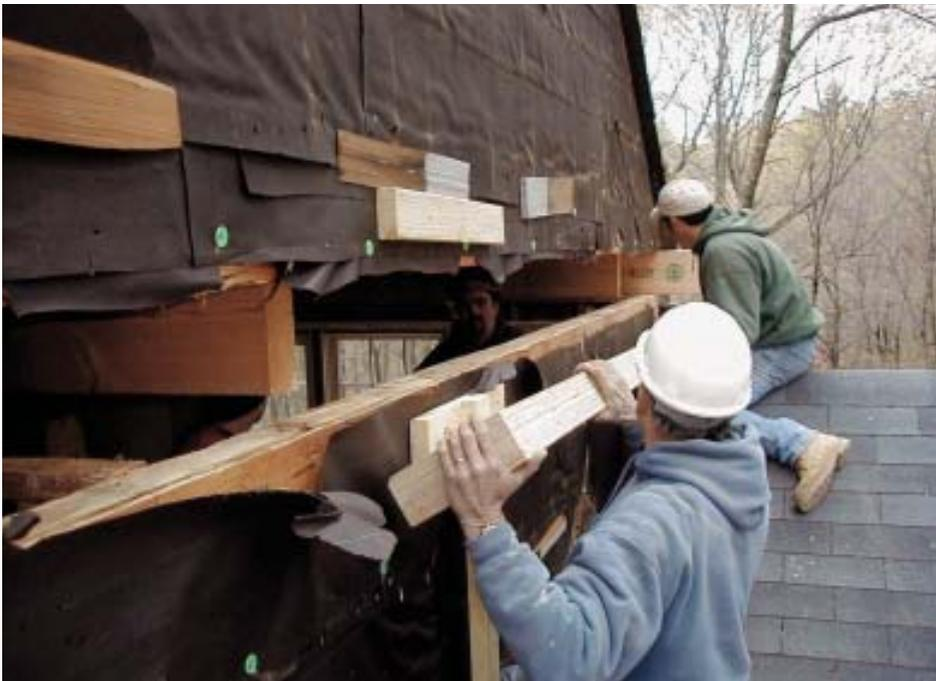
**Figure 4.** Working in small increments, the seven-man crew slowly raised the roof structure by 9 $\frac{1}{2}$  inches, allowing the nominal 4x10 engineered LVL plates to be inserted into position on top of the wall.
