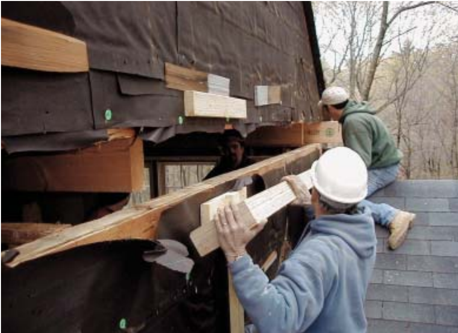
Figure 4. Working in small increments, the seven-man crew slowly raised the roof structure by 9½ inches, allowing the nominal 4x10 engineered LVL plates to be inserted into position on top of the wall.
