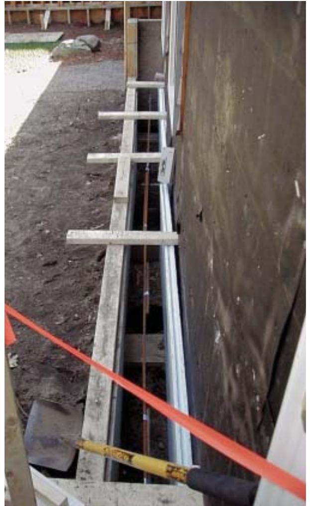
piers placed every 4 to 5 feet. We reinforced the piers vertically with rerod bent at right angles to join the horizontal rerod we placed in the grade beam.
