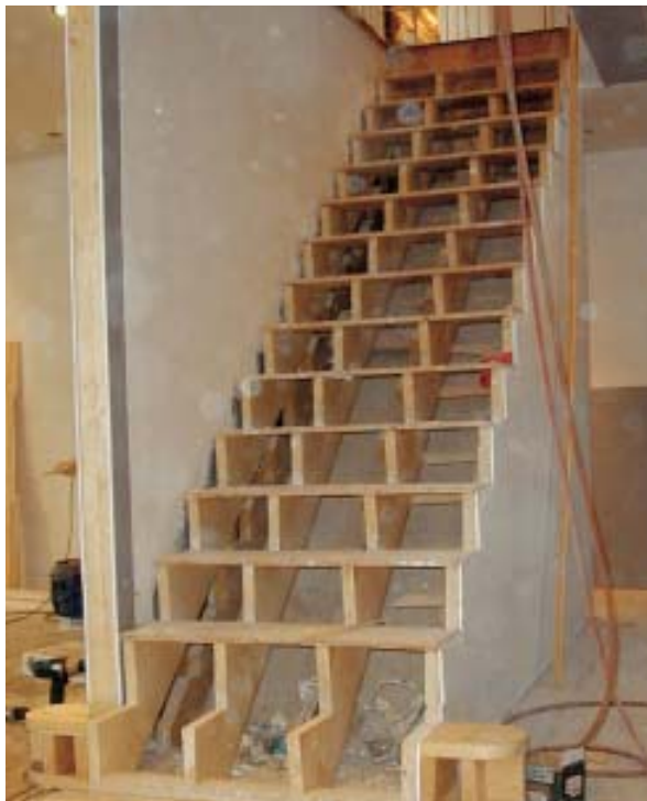
Figure 6. Though the staircase would be rebuilt, the original stair helped determine the distance that the first-floor ceilings were raised: two riser heights, or 15 inches.
