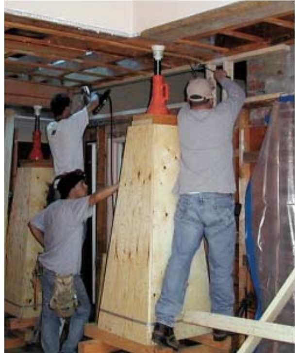
Figure 10. While the front wall went up quickly to support the building at its new height (left), the center and rear partitions had to be revised one stud at a time, by cutting and sistering in full-length studs under a new top plate. Nonbearing interior partitions were elevated with short cripple-wall sections (below).
